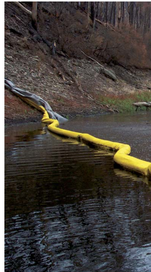
Managing our supply for uncertainties. Bendora Dam after the January 2003 bushfires. A boom and curtain are in place to reduce sediment impacts.
