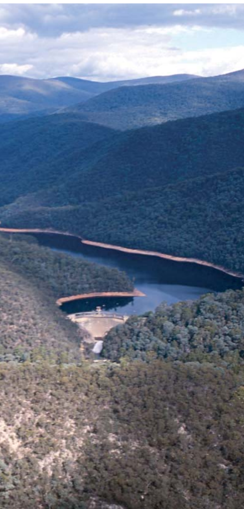
Bendora Dam before the January 2003 bushfires. This pristine catchment has traditionally been the preferred supply for Canberra's drinking water.
